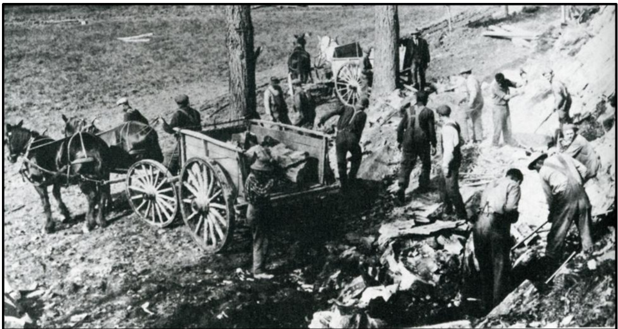
Perini employees working on the Cochituate Reservoir
